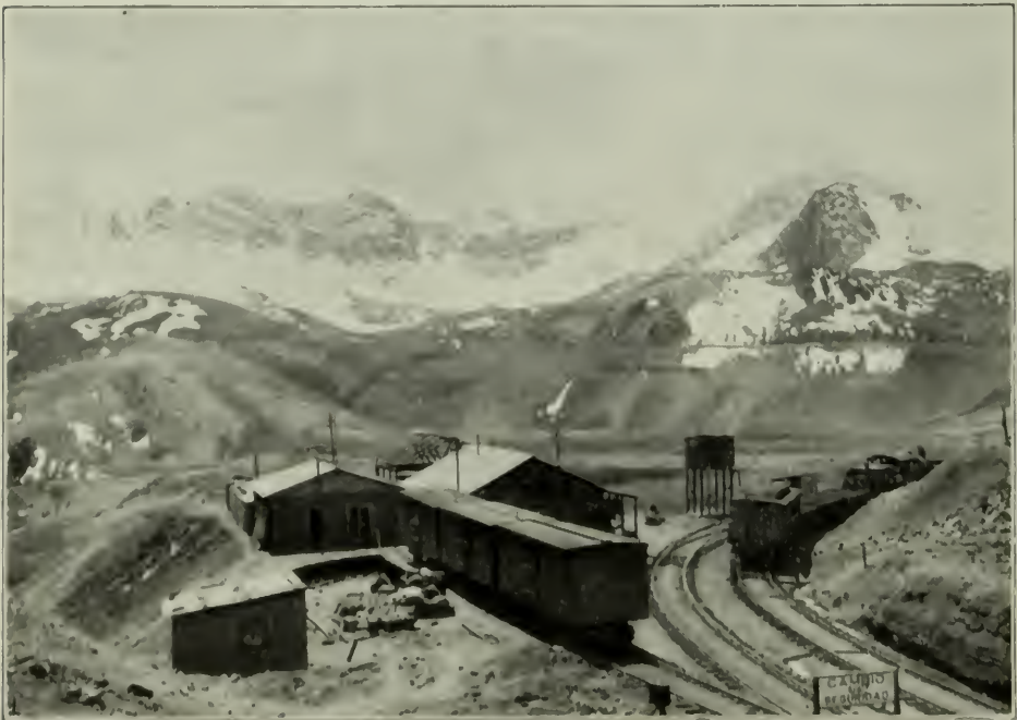
TICLIO, ON THE PERU CENTRAL RAILWAY, THE HIGHEST TELEGRAPH STATION IN THE WORLD.
